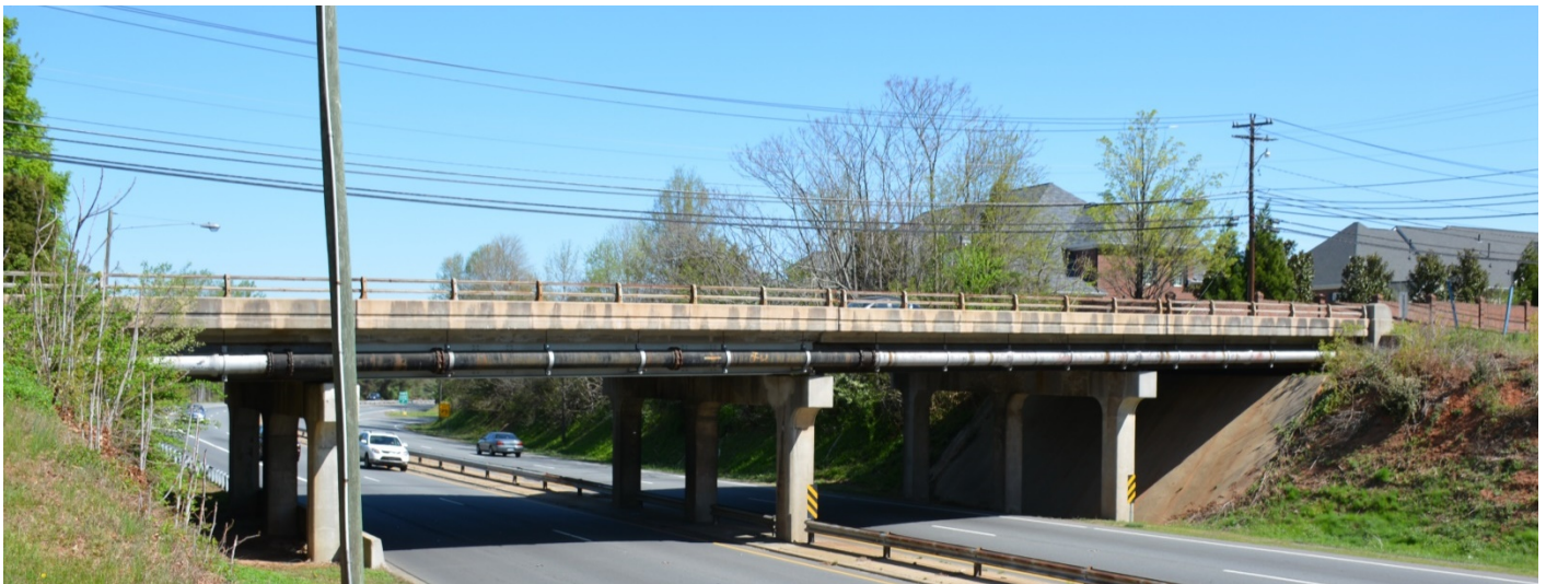
Bridge No. 276 over Silas Creek Parkway
