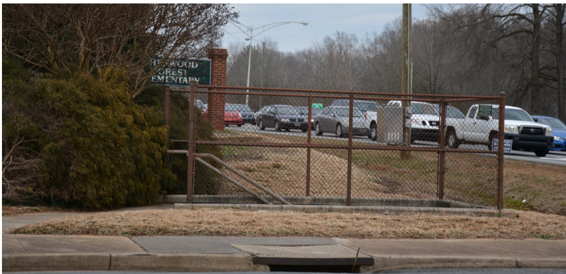
Pedestrian tunnel at Silas Creek Parkway and Yorkshire Road's intersection, looking north
