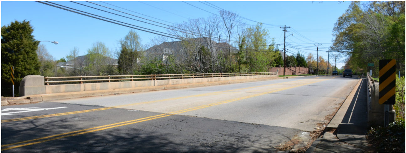
Bridge No. 276 looking east on Country Club Road
