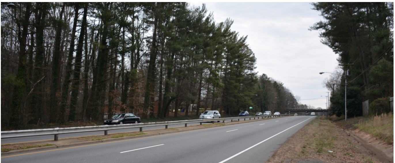
Silas Creek Parkway looking north toward Country Club Road bridge
