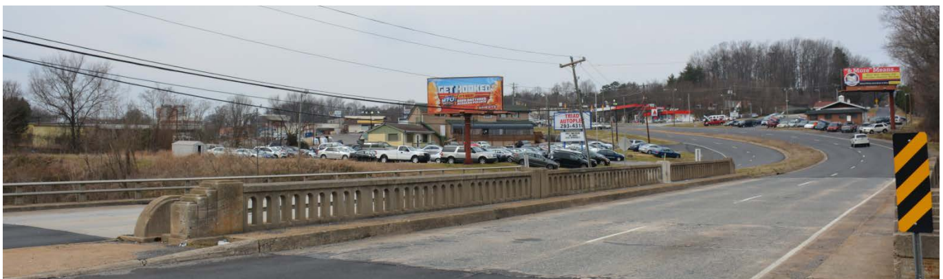
Silas Creek Parkway looking west at bridges over Salem Creek
