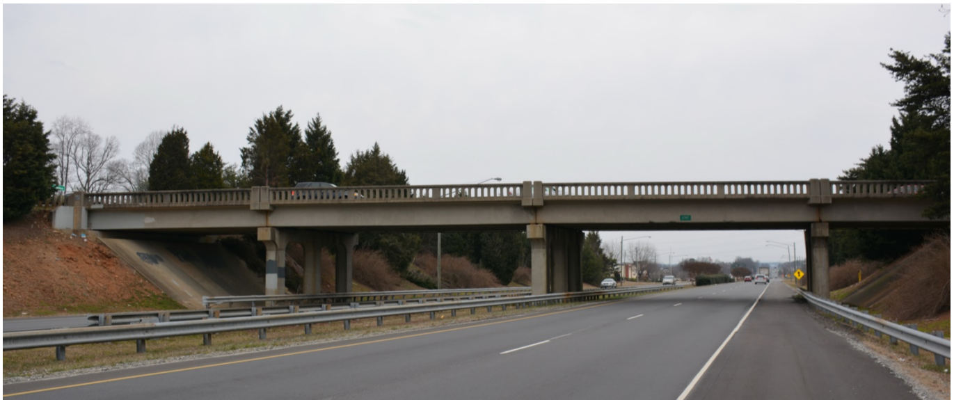
Peters Creek Parkway looking north at the Clemmonsville Road Bridge
